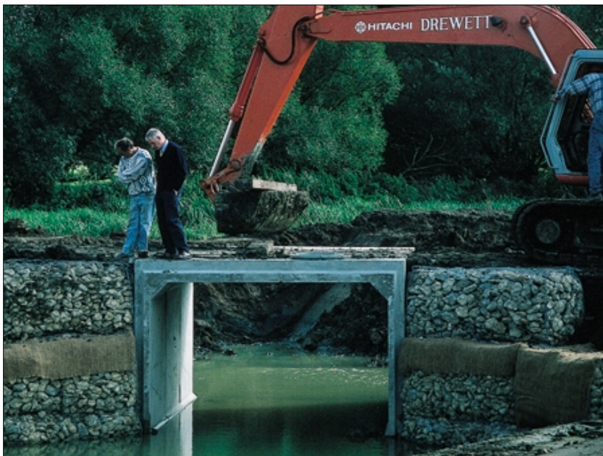
New concrete culvert crossing under construction
