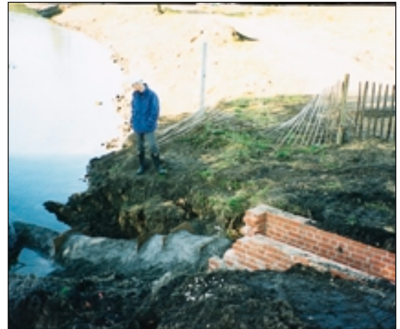
New outfall chamber under construction
