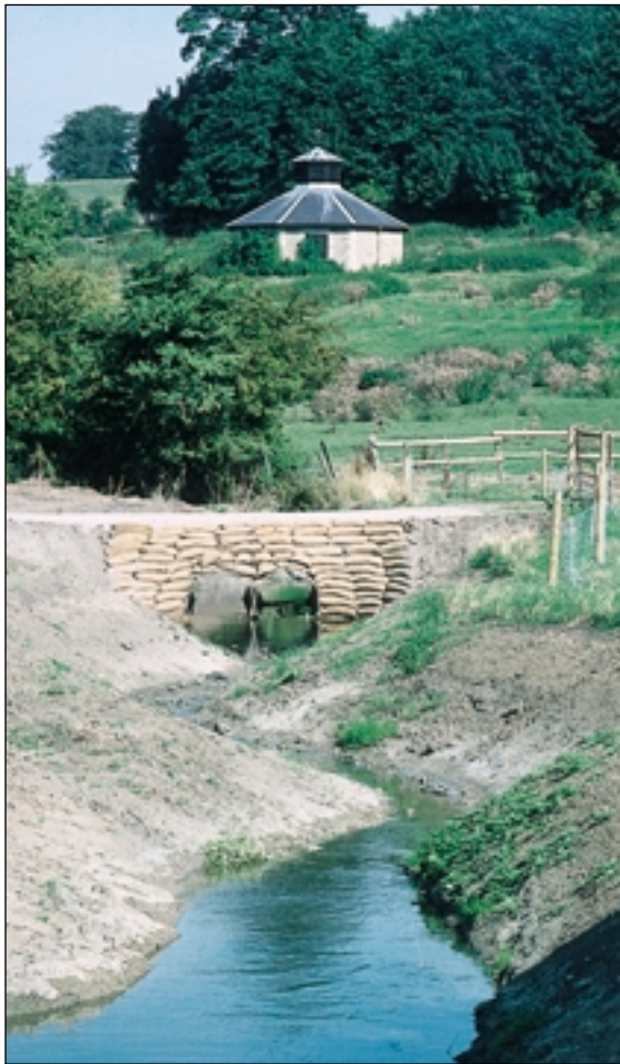
Flood drain crossing seen from bank of R. Cole. (bagwork wing walls incomplete)
