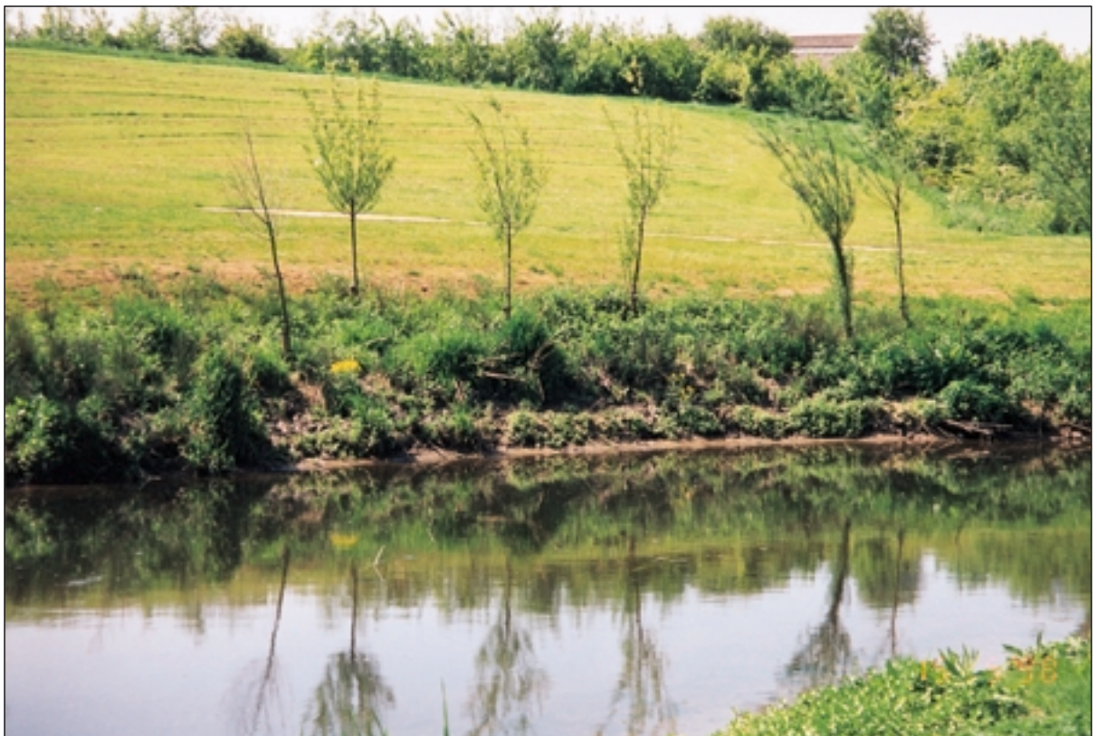
Slipped slope 2 years after repair – 1997
