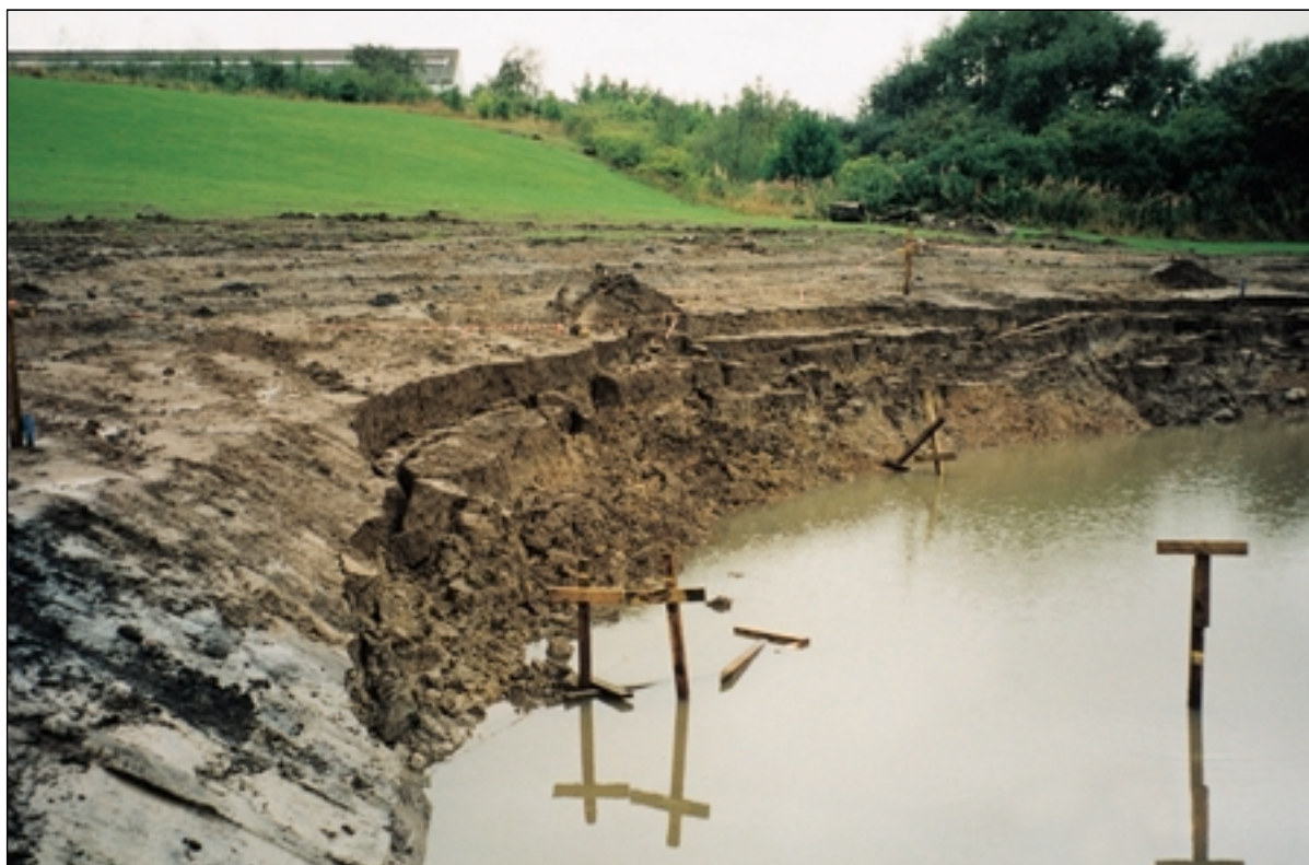
Slipped slope during work – September 1995
