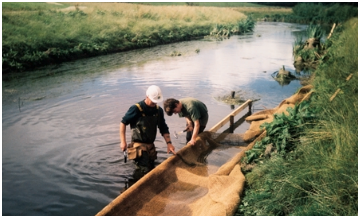
Attaching coir matting to create Type A ledges on River Skerne
